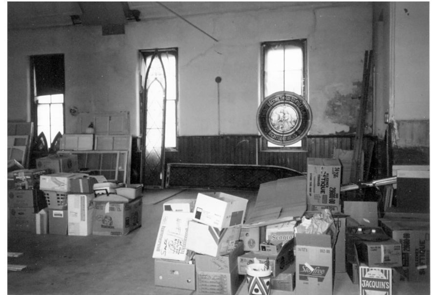
CMCL SANCTUARY BEFORE RENOVATION
